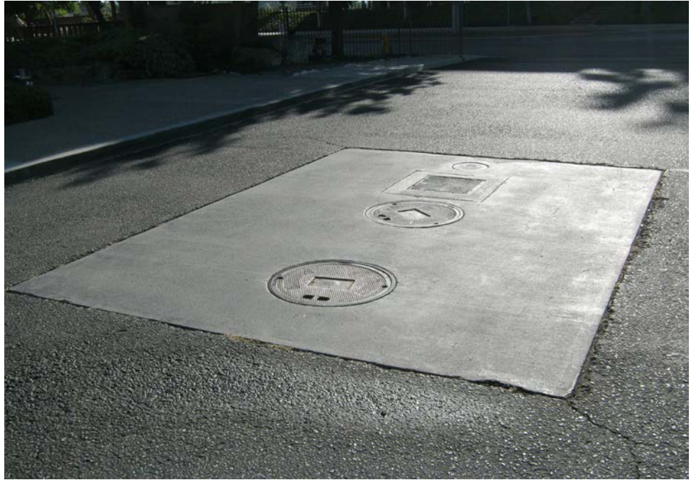
Photograph 3: View of clarifier southwest of the site building.
