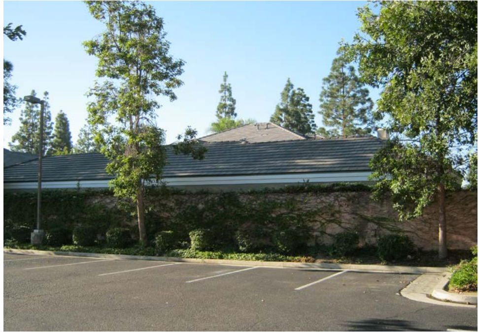
Photograph 13: Looking southwest at the site, beyond which are residential properties.
