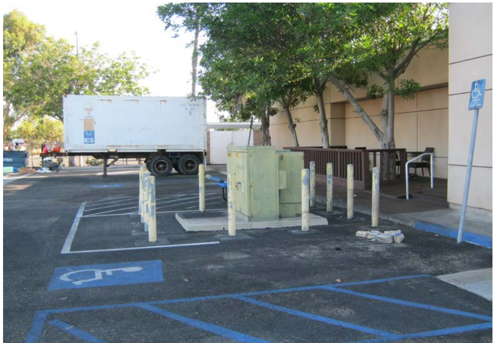
Photograph 4: View of pad-mounted transformer northeast of the site building.
