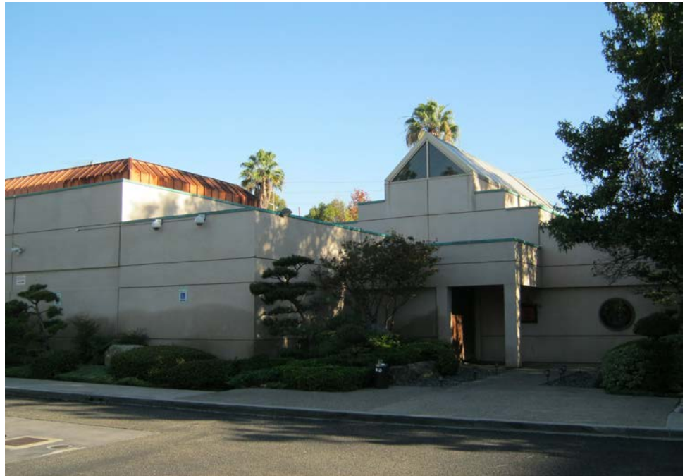
Photograph 1: Looking northeast at the site building.
